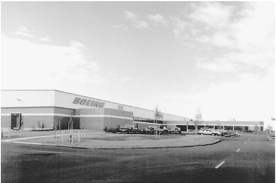
FIGURE 1.9 A large manufacturing facility housed in a pre-engineered building. (Photo: Varco-Pruden Buildings.)
