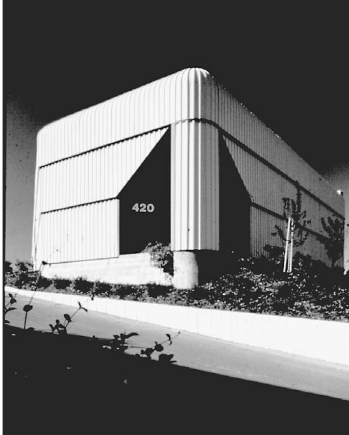
FIGURE 1.7 A modern manufacturing facility made possible with metal building systems. (Photo: Bob Cary Construction.)
